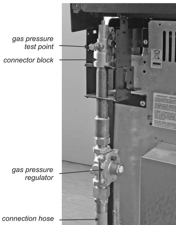
Because the height of the cooker can be adjusted and each connection is different it is difficult to give precise dimensions. Ideally the house supply connection should be in the shaded area shown in the diagram. Means of isolation must be provided at the supply point by either an approved quick-connect device or a Type 1 manual shut-off valve. The hose should be fitted so that both inlet and outlet connections are vertical so that the hose hangs downwards in a 'U' shape.
